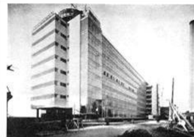
49. Van Natta Factory, Rotterdam, by Van der Vlugt and Brinkman. 1928
