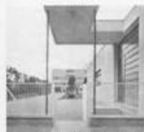
46. Study and entrance house of the University, Garden (Holland) by J. van der Vlugt. 1901-1902
