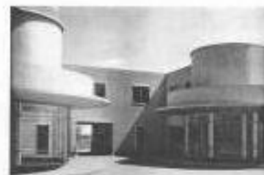
47. Study and entrance house of the University, Garden (Holland) by J. van der Vlugt. 1901-1902
