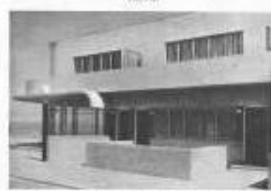
48. Study and entrance house of the University, Garden (Holland) by J. van der Vlugt. 1901-1902
